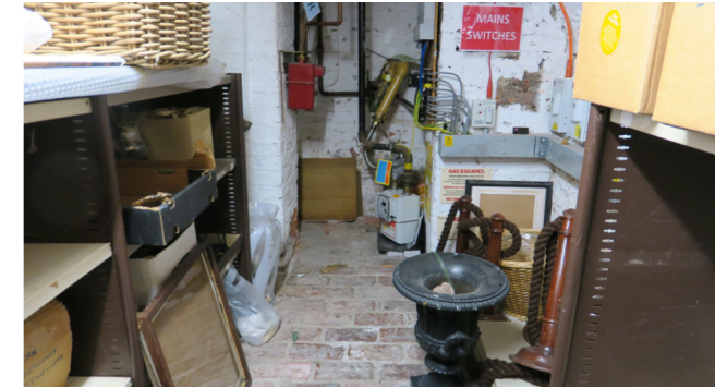
West Cellar, South Elevation
