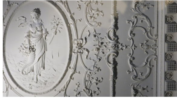
Stucco Ceiling Detail
