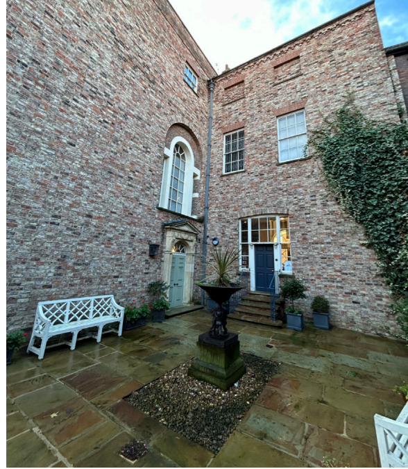
North Elevation, viewed from first floor landing.
