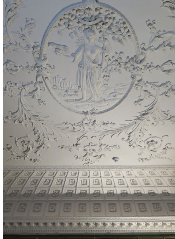
Stucco Ceiling Detail
