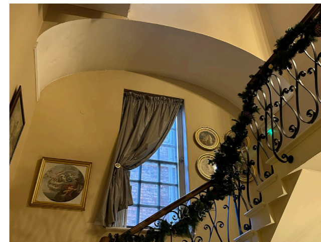
East elevation, window on half landing between ground to first floor.
