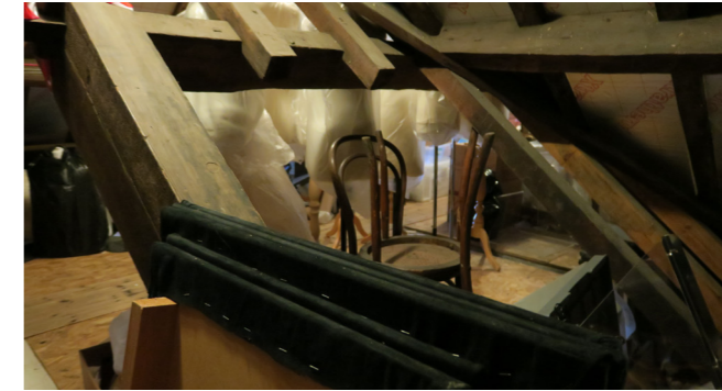
Attic 2, South-West view from head of stairs.
