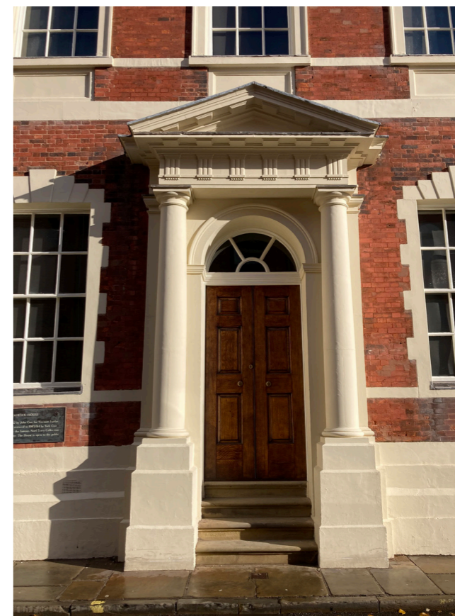
South Elevation, main entrance door off Castlegate
