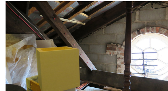
Attic 2, South Elevation.
