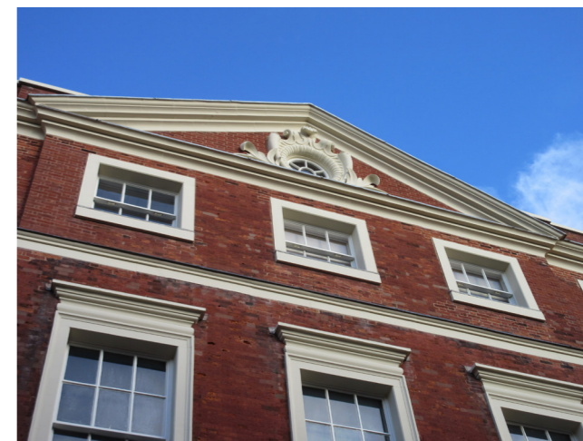
South Elevation, looking up to top floor frontage of No.27.
