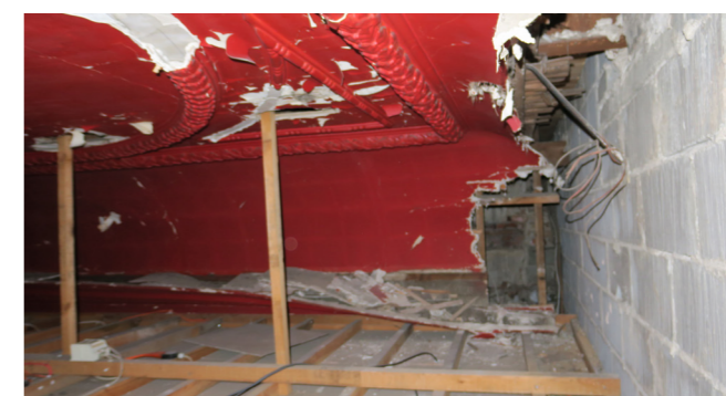
Concealed Stucco Roof above Suspended Ceiling.
