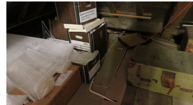
Attic 2, York Civic Trust use the space to store varying administrative and Archival materials.
