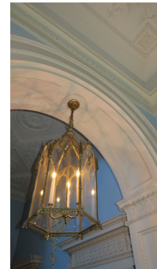
South Elevation; North arch detail.
