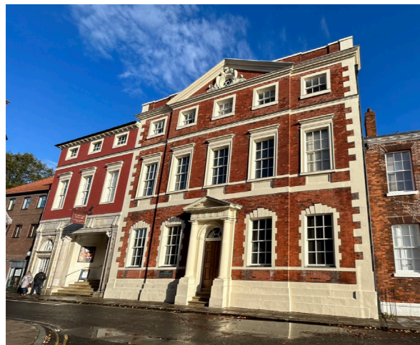
Principal Elevation facing Castlegate
