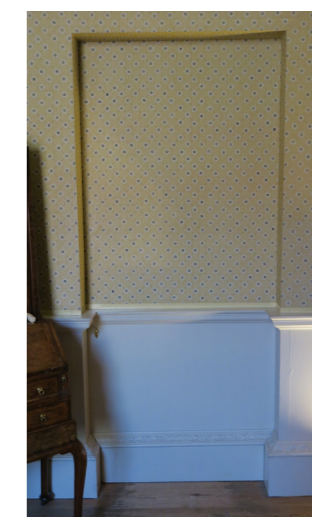
Cornice Detail; Modern jib door formed 1982-4.
