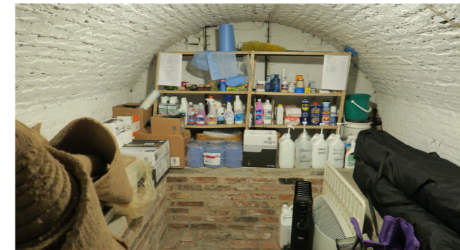
Middle Cellar, South Elevation
