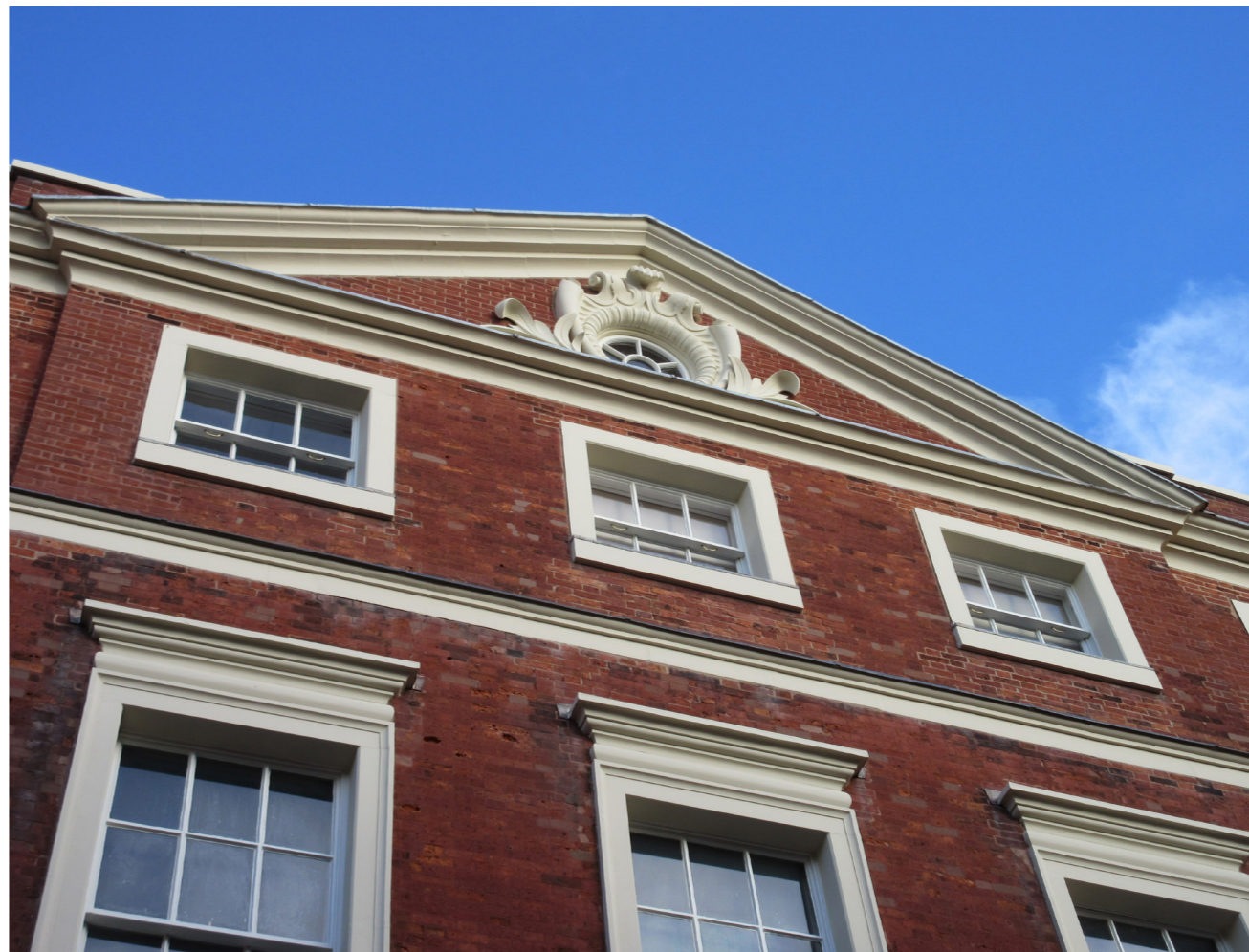
Looking up to existing frontage from Castlegate Street below.
