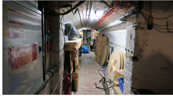
South view at stair base.
