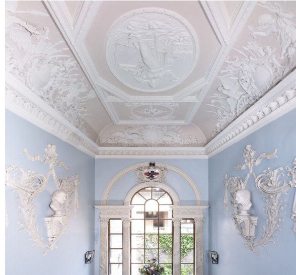
West window and ceiling detail, from first floor landing.
