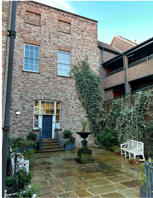
Left to Right - North-west Courtyard; North- East return Elevation (above Rear Stair Hall Entrance); North Approach Stair; Ground Floor WC Elevation (North).
