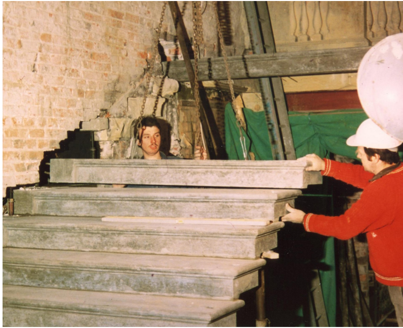
Replicating the lower rear staircase, c.1982-4. York Civic Trust Archive.
