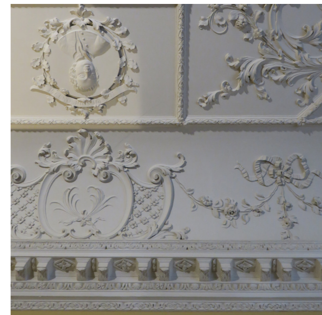
Ceiling Cornice Detail
