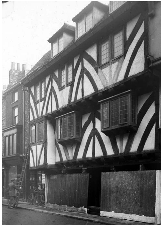
Fig. 5.14 Photograph of 1929 showing the restoration in progress. The pale replacement oak timbers can be clearly seen © City of York Archives.
