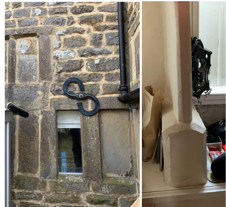
Figure 5.5 Left - Mullion windows on rear elevation of Brereton House, including blocked c.1740 stair light (top left) with later light inserted below (now also partially blocked). Right - detail of the interior mullions.
