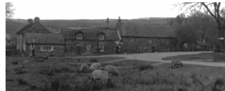
Figure 5.12 Photograph of 1955 showing the insertion of two dormer windows into the roof of Brereton Cottage, and alterations to Brereton Corner © Frincis Frith.
