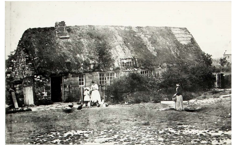
Figure 4.2 High Mortar Pit Cottage, Goathland, with heather-thatch roofing - late C19th photo. Now demolished, High Mortar Pit was located to the immediate west of Brereton © North Yorkshire & Cleveland Vernacular Buildings Study Group H342.
