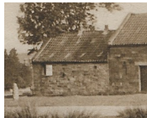
Figure 5.13 Detail from undated early C20th postcard showing Brereton Corner cowhouse with a single shuttered window and pantile roof.
